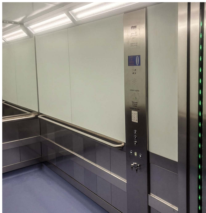
Lift car with new finishes, car operating control panel
