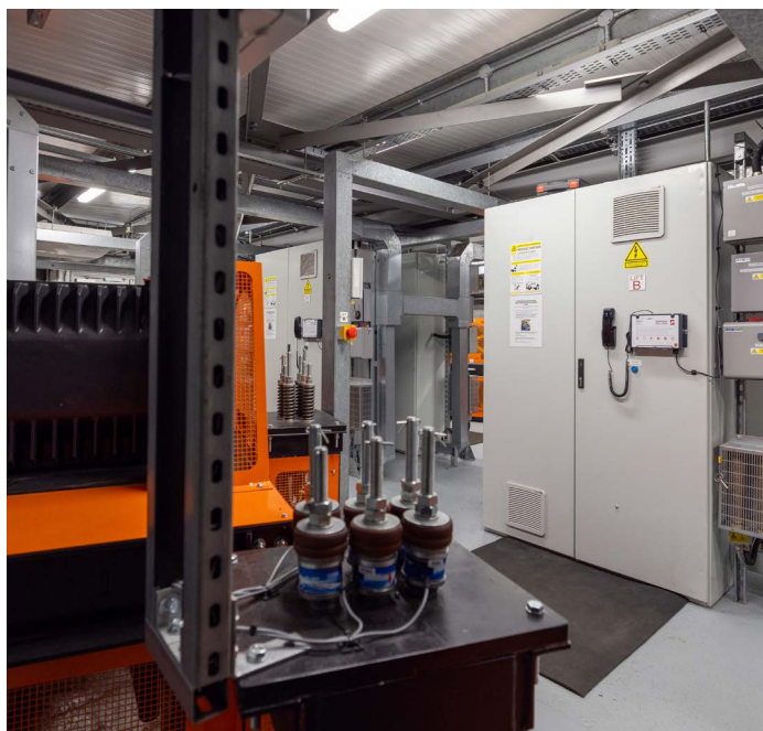
Lift controller cabinets
