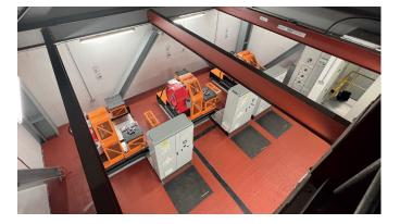
assist with the movement of goods in the building. The modernisation of all six lifts included the installation of new J&L high-speed gearless machines, Kollmorgen lift controllers, new auto-diallers, shaft safety gear, new landing and car doors, car operating panels and landing signalisation.
