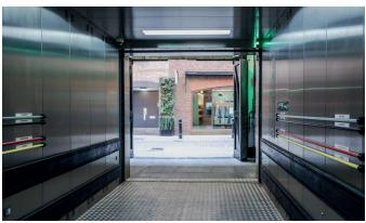
the lift car. The decision was also made to include heavy-duty vertical sliding lift doors at both ends of the lift car. This would allow for cars to move through the lift and into a parking bay.
