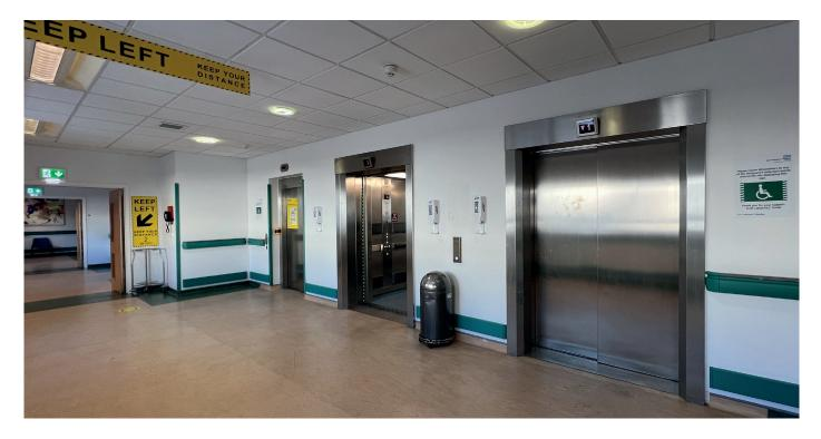
This included the dismantling and removal of the old equipment and the installation of new drives, lift controllers, shaft wring, new lift car and doors, full car relines, car operating panels and landing signalisation. Jackson also undertook a new installation of a duplex pair of bed lifts, again serving the Hospital's three floors.
