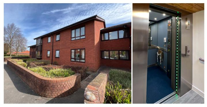
The modernisation included a new hydraulic valve and lift control system. Additionally, we also installed new landing and car signalisation, shaft wiring and lift positioning equipment (limits). One of the key benefits for residents has been better floor levelling, whilst at the same time, achieving our customer's secondary objective of improved energy efficiency.
