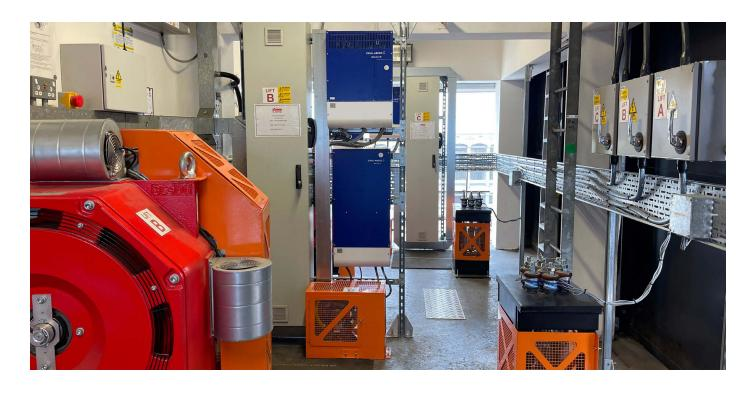
The decision was made to install compact highspeed, gearless drives and new fully collective lift controllers to work as a group of six lifts under a destination control system. We also undertook a full modernisation of the car and landing doors, lift shaft equipment and re-roped each of the six passenger lifts.
