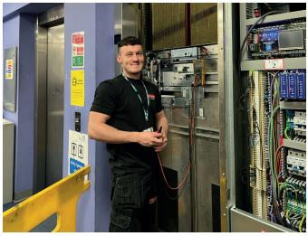
In consultation with the Trust, Jackson proposed the replacement of the troublesome equipment, which included the lift controllers and door gear. With the Trust's agreement, we commenced with a modernisation programme for each lift. Due to social distancing requirements being lifted, the building was fully occupied and our local engineers worked on one lift at a time to ensure continuous lift availability.
