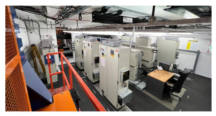
for refurbishment and subsequent reinstallation. The remaining lifts comprise of two firefighting and one goods lift which serves eleven floors, all three had new machines installed as part of the modernisation project.
